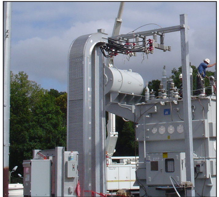
MP Husky 4000Amp, 5kV Cable Bus System with open air termination to GSU transformer.
